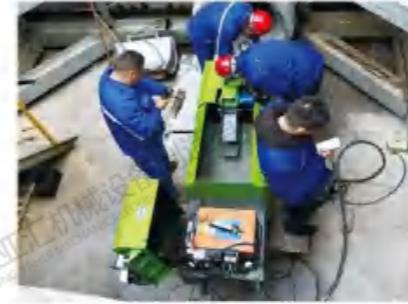
管道清渣小车 Pipeline slag removal trolley
